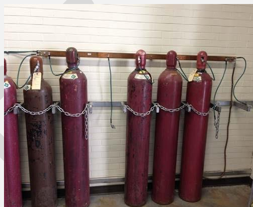
COMPRESSED GAS CYLINDER STORAGE AREA. (Figure – 6)
